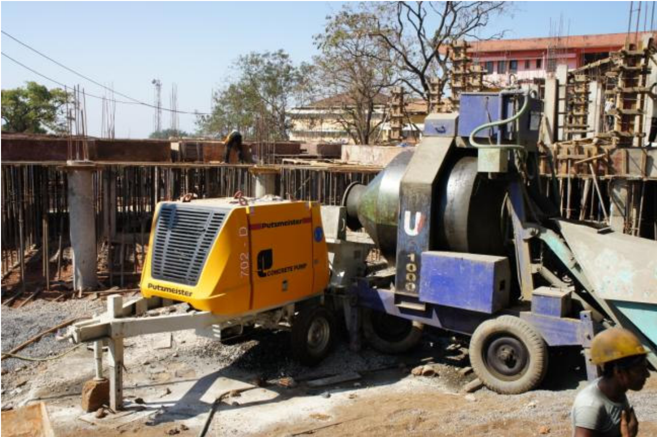
BSA 702D working at the Construction site of Govt. Medical College, Goa
