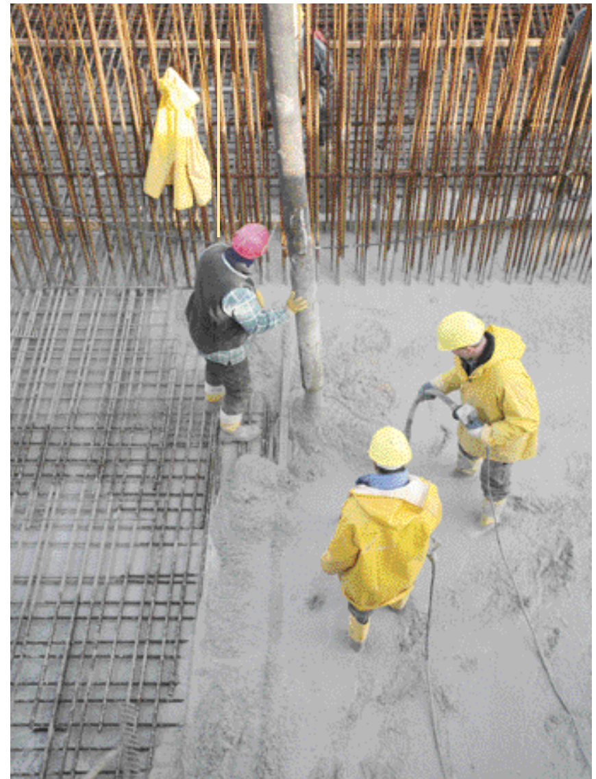
Fig. 9: Compacting the concrete with vibrating cylinder
