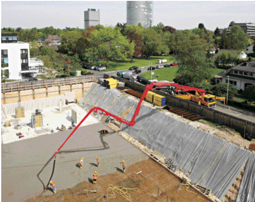
Fig. 1: Putzmeister M 42-5 truck-mounted concrete pump in Bonn
