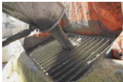
Fig. 20: Pumping of high-density concrete in compressive strength class C100/115
